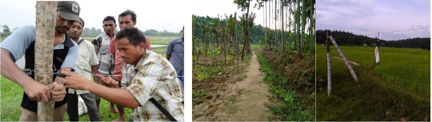
Community fencing being erected at WB Fencing erected at Kerala (Vengoor, Athikunni, Kalankandy)
